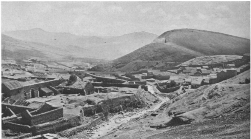
FIG. 6—Looking down the Ribera; masonry canal (left of center) for turning water wheel.
