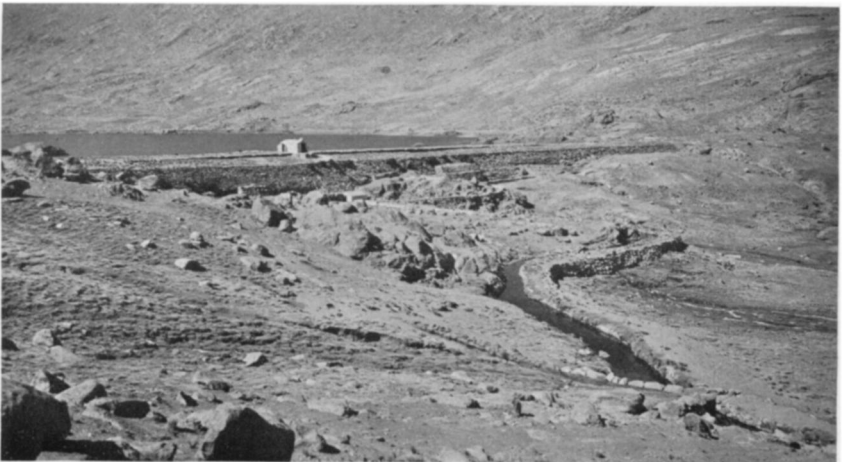
FIG. 18—Looking upstream toward Chalviri dam and outlet canal.
