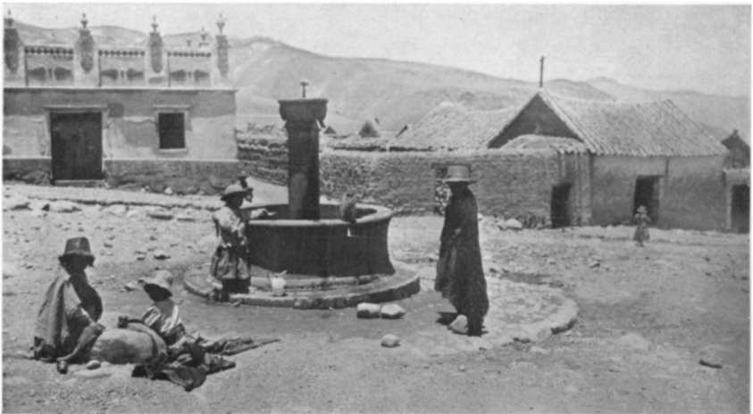
FIG. 4—One of the pilas where the people of Potosí go for water.
