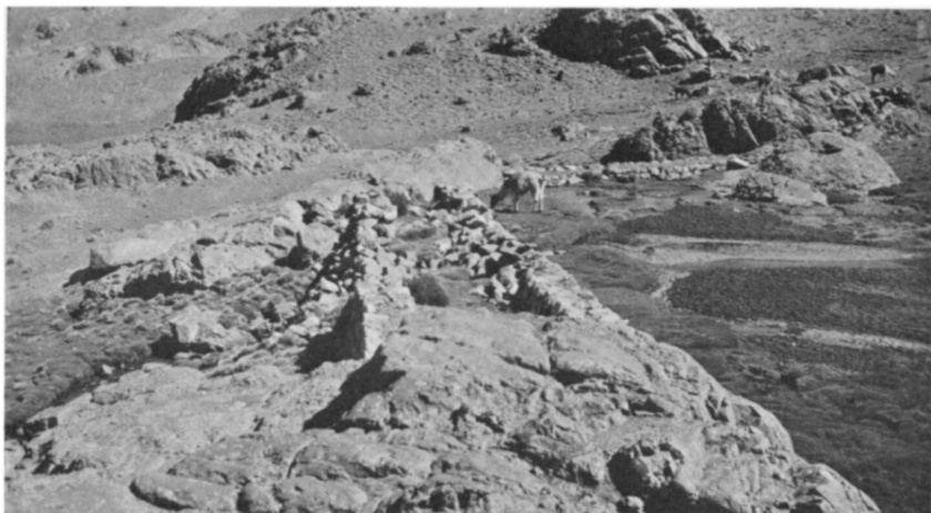
FIG. 20—Remains of dam of "lost" lake found by the writer in the Soras quebrada in 1935, and now put into service.
