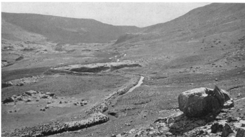
FIG. 19—The Chalviri aqueduct.
